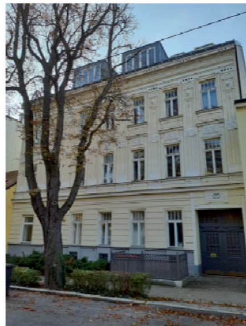
Figure 2. The demonstration project in Iglaseegasse is a typical Gründerzeit style house in Vienna.
